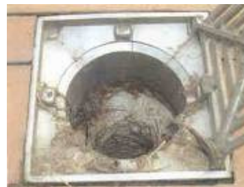
Efflorescence directed to the drain
