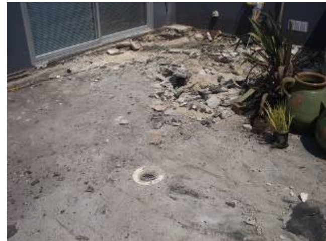
Remove saturated screed to get back to slab or primary structure
