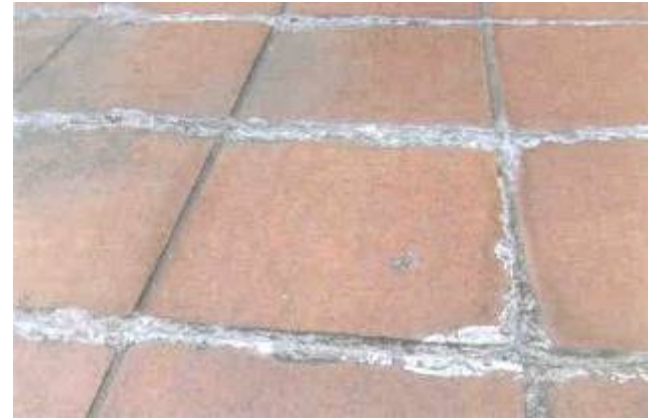
Typical efflorescence in mortar joints from saturated screed
