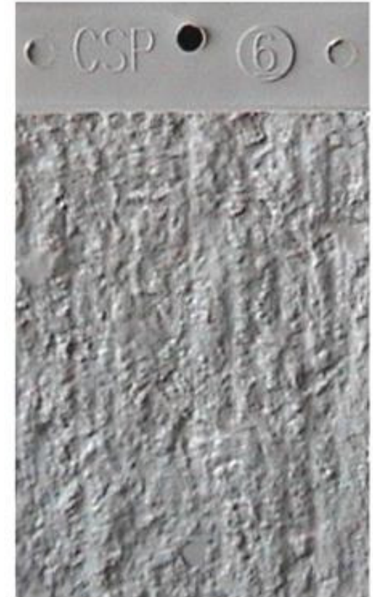
CSP 6 Medium scarification
