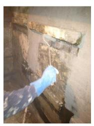
Most occasions in which Negative Tanking occurs is due to remedial action. Either structural damage has occurred, the membrane system has failed or no waterproofing was installed. In some occasions the water problems are not solved, but the situation managed.
