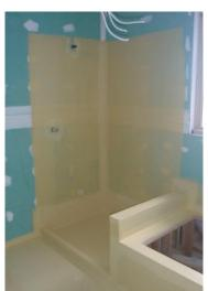
Floor preparation may require grinding, installation of Hobs and Water Stops. Some floors also require a vapour barrier application before applying a waterproofing membrane. Options for decorative wear surfaces typically include tiles or epoxy coatings.
